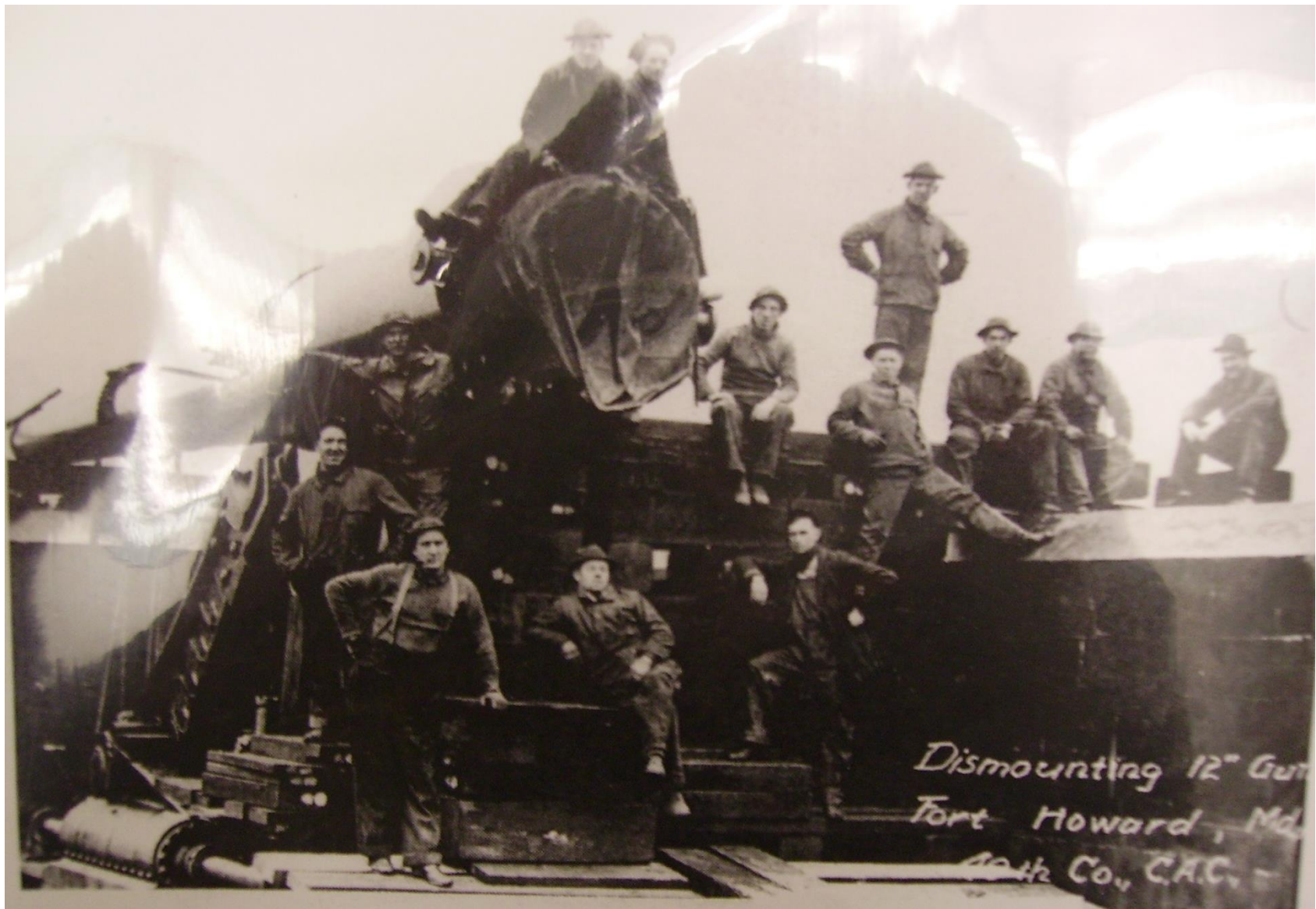
1917 - A picture of the 40 th company dismounting one of the 12-inch rifles. The guns were suppose to be sent to France and used against the Germans during WWI but we're not sure if they made it before the war ended in 1918.
