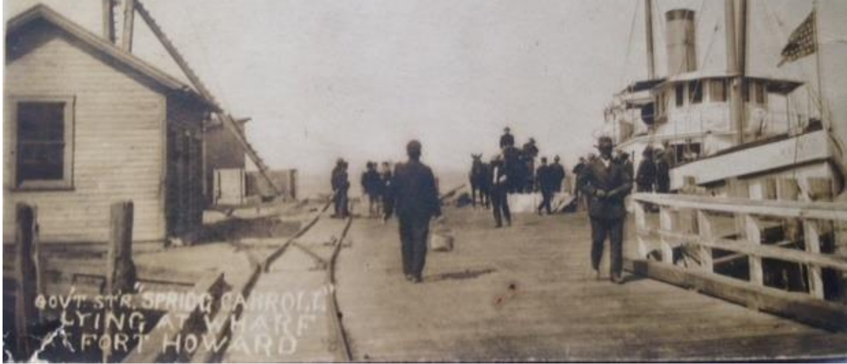
Another post card from 1907. This is a view of the far end of the (900 foot) pier. The ship on the right is the ferry "Sprigg Carroll". Note the railroad tracks. A small steam train moved supplies from the boats into the fort and carried the underwater mines from storage out to the mine tender boat.
