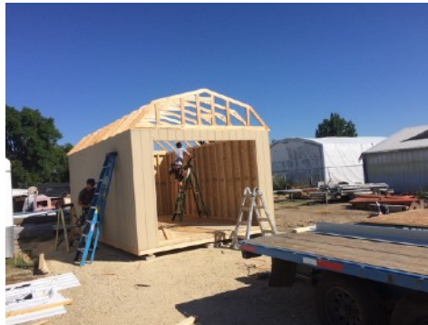
Rafters and siding on.
