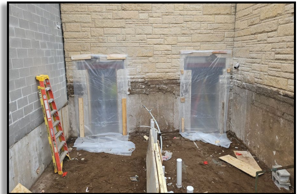
Doors Cut Into Existing Gym
