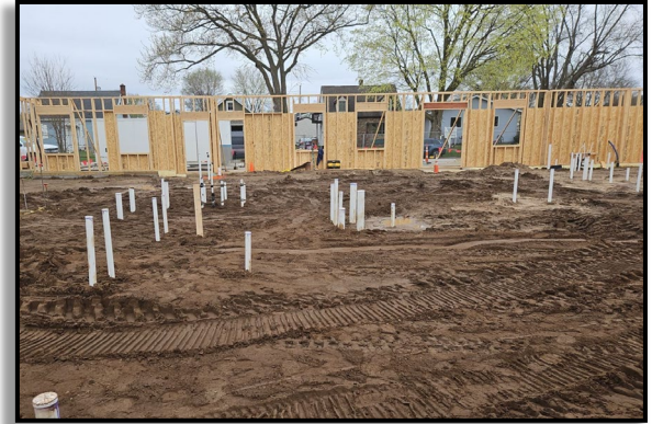
Electrical & Plumbing Underground
