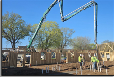
Pouring Interior Concrete Footings
