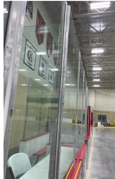
#18 Dasher boards leaning into, and back of rink.
