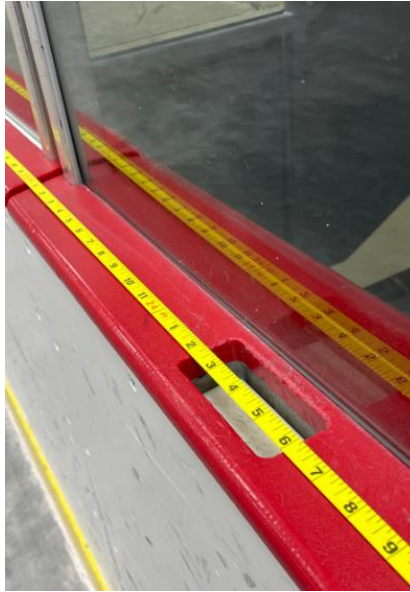
#24 Access Gate push button sticks (loose fasteners).
