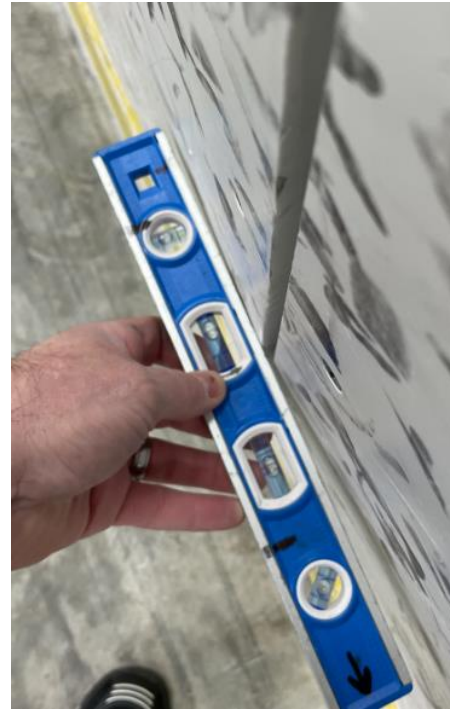
#28 Board bent from Zam hit.
