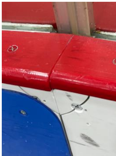
#22 Cracked facing at seams in multiple locations
