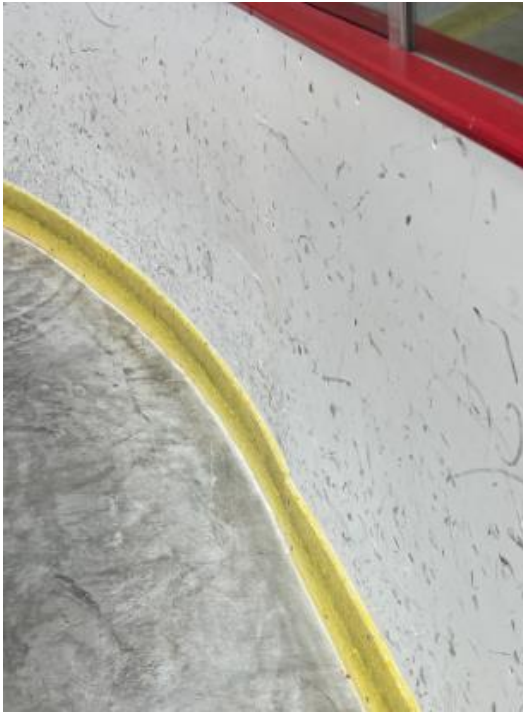
#27 Board bent from Zam hit.
