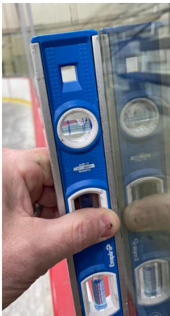
#25 Glass Leaning into rink.
