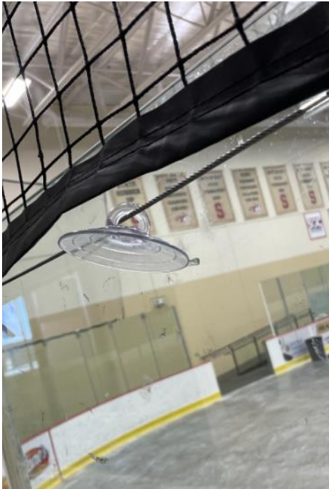
#32 Suction cups not attached.
