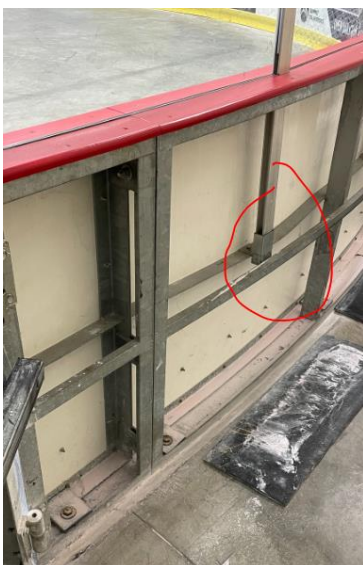
#29 Board bent from Zam hit.
