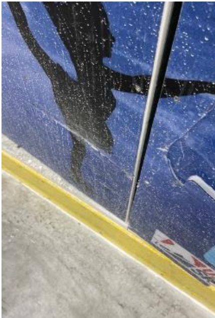
#5 Players gate hit with Zam. Frame bent.
