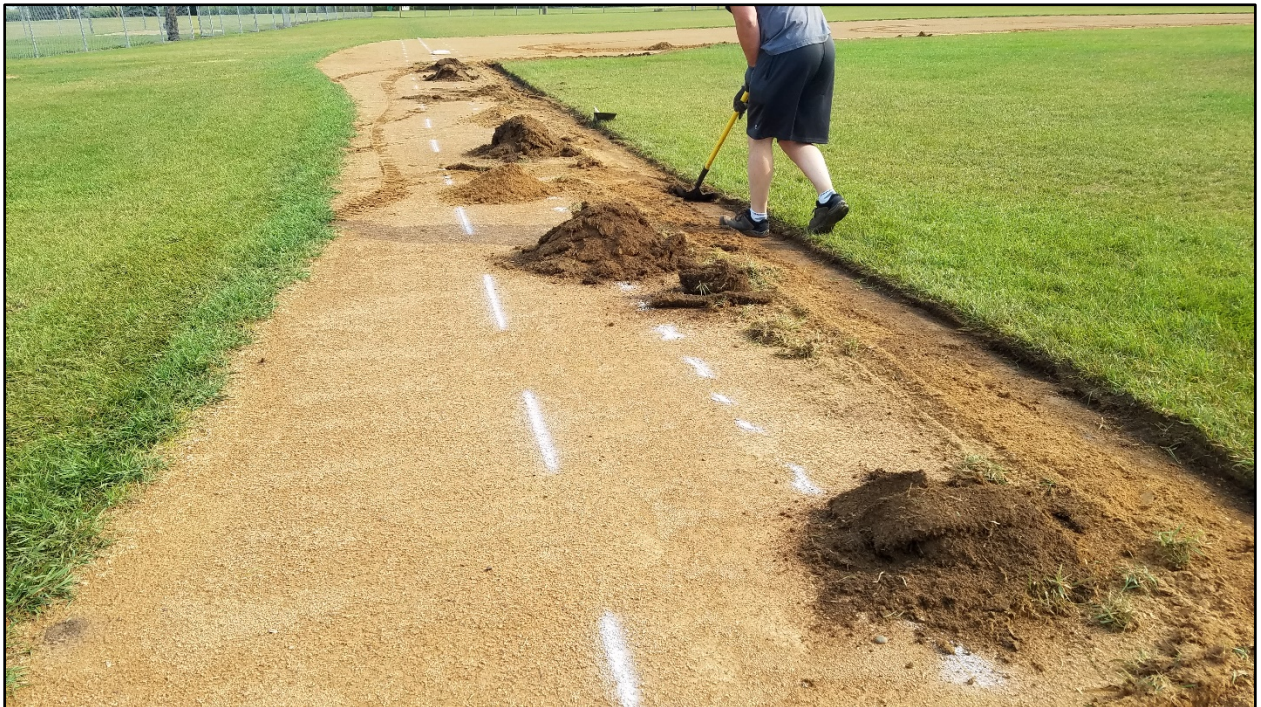
Sod-lines cut using motorized sod-cutter and hand tools.
