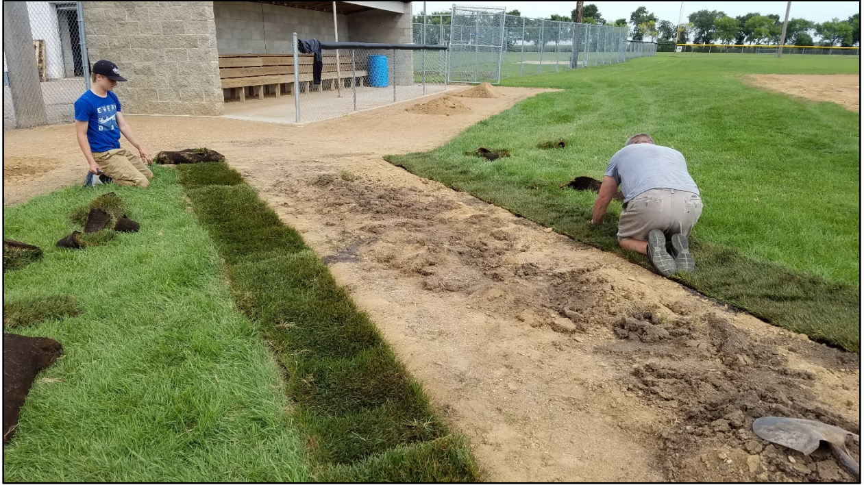
Dugout to home plate walkways were cut and brought back to standard dimensions. New sod laid.
