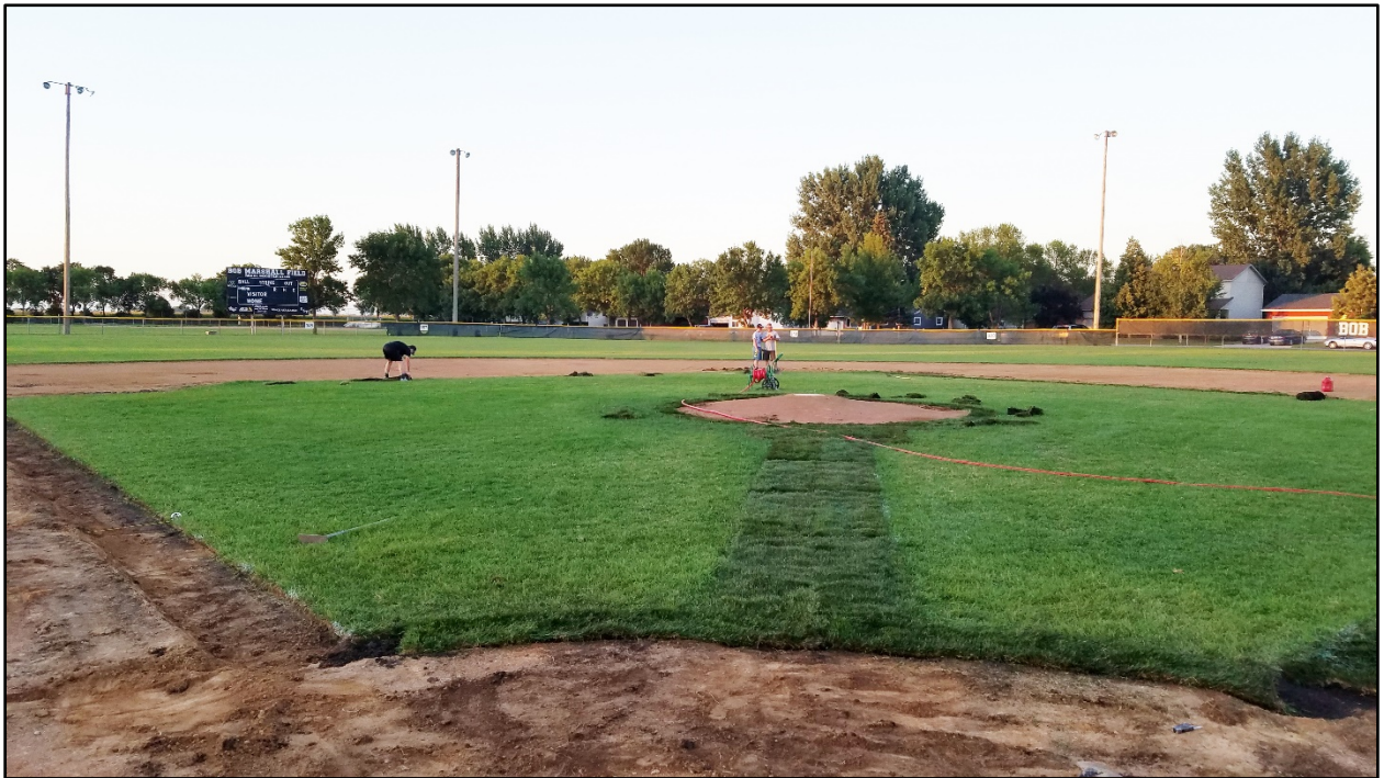
All infield sod-lines were cut straight, leveled and re-sodded. The mound to home plate dirt path was filled in with new sod.
